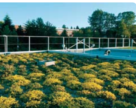
The roof of the Green Roof Research Facility at BCIT Centre for Architectural Ecology in Burnaby.
